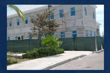
Phase I of the project, encompassing the installation of structural components including foundations, substructures, interior/exterior load bearing walls, roofing and exterior doors and windows, was completed in December 2015. Work also continued on the exterior façade to maintain uniformity with the rest of the campus facilities. Once completed, the centre will serve as a beacon for higher education and graduate scholarship in the country.
