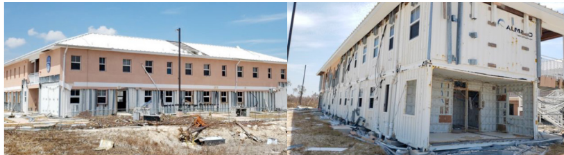
Figure 9: The Damaged Main Building and Dormitory on the University Campus.
