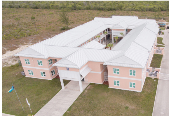
Figure 8: Aerial View of UB-North Prior to Hurricane Dorian.
